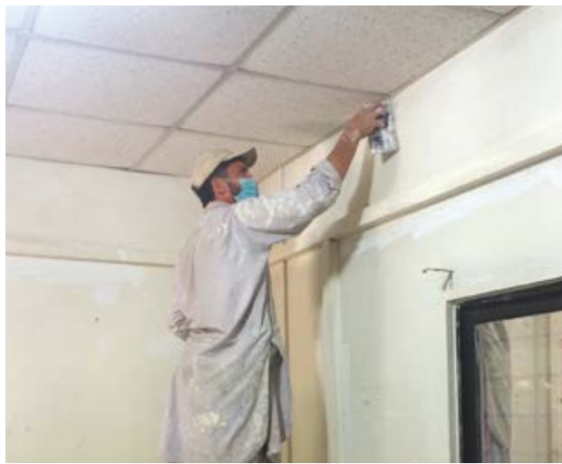
Field Station Rawalakot under renovation.
