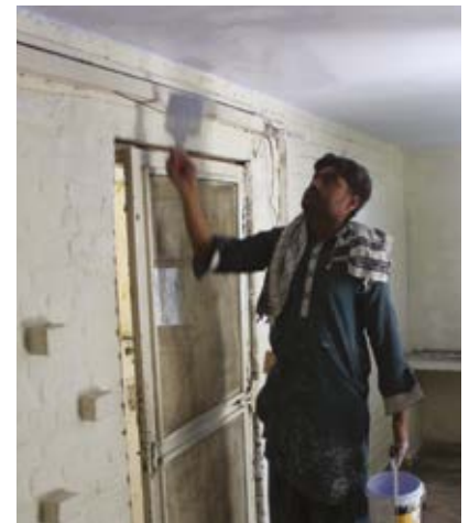
Field Station Bhimber under renovation.
